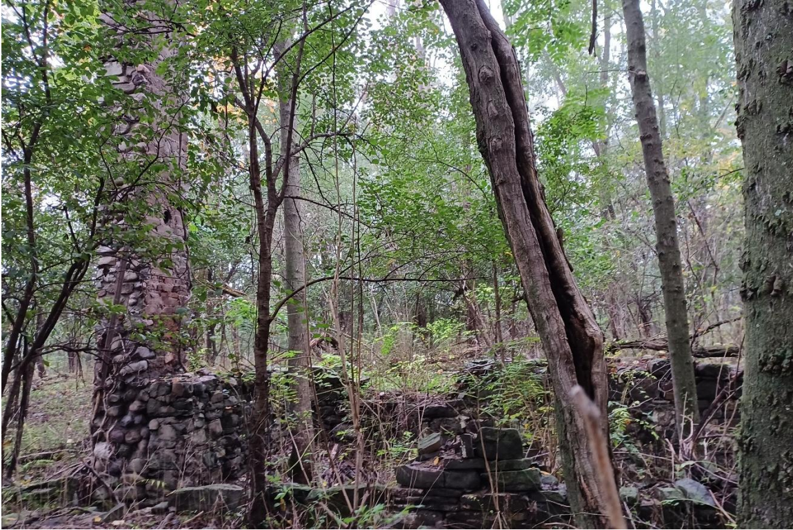
Photo 23: The foundation for the residential structure (F2) features modern concrete and a gutter on the outside of the chimney. View to the southwest.
