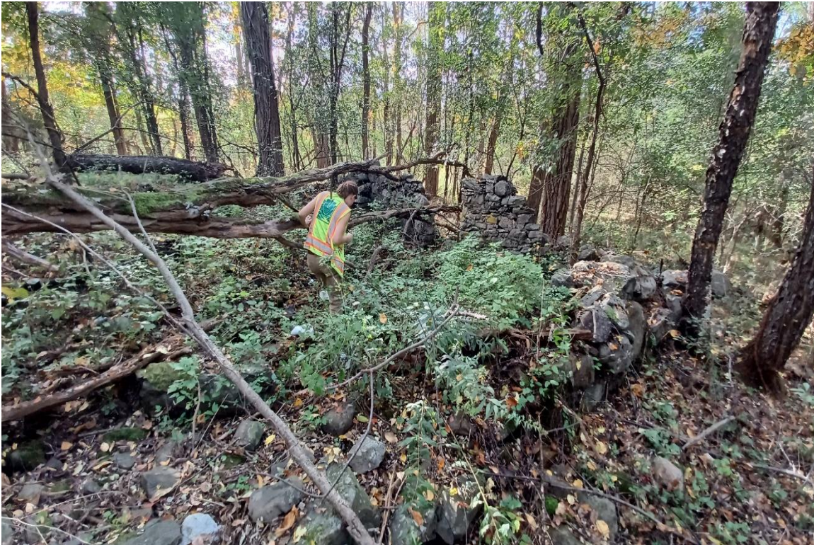
Photo 10: The stone foundations in the eastern portion of the APE are primarily collapsed ruins of a residential structure and barns. View to the northeast of F2.
