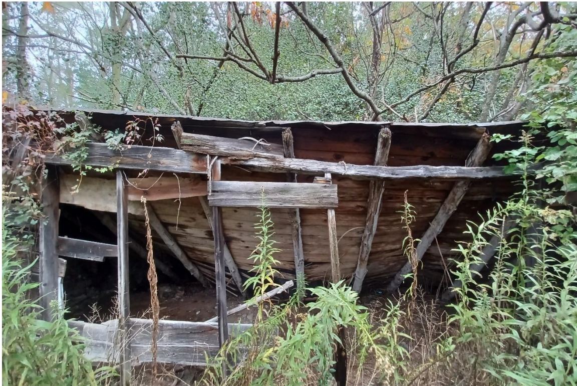
Photo 24: The 3-sided barn (F3) has been constructed with twentieth century materials. View to the north.
