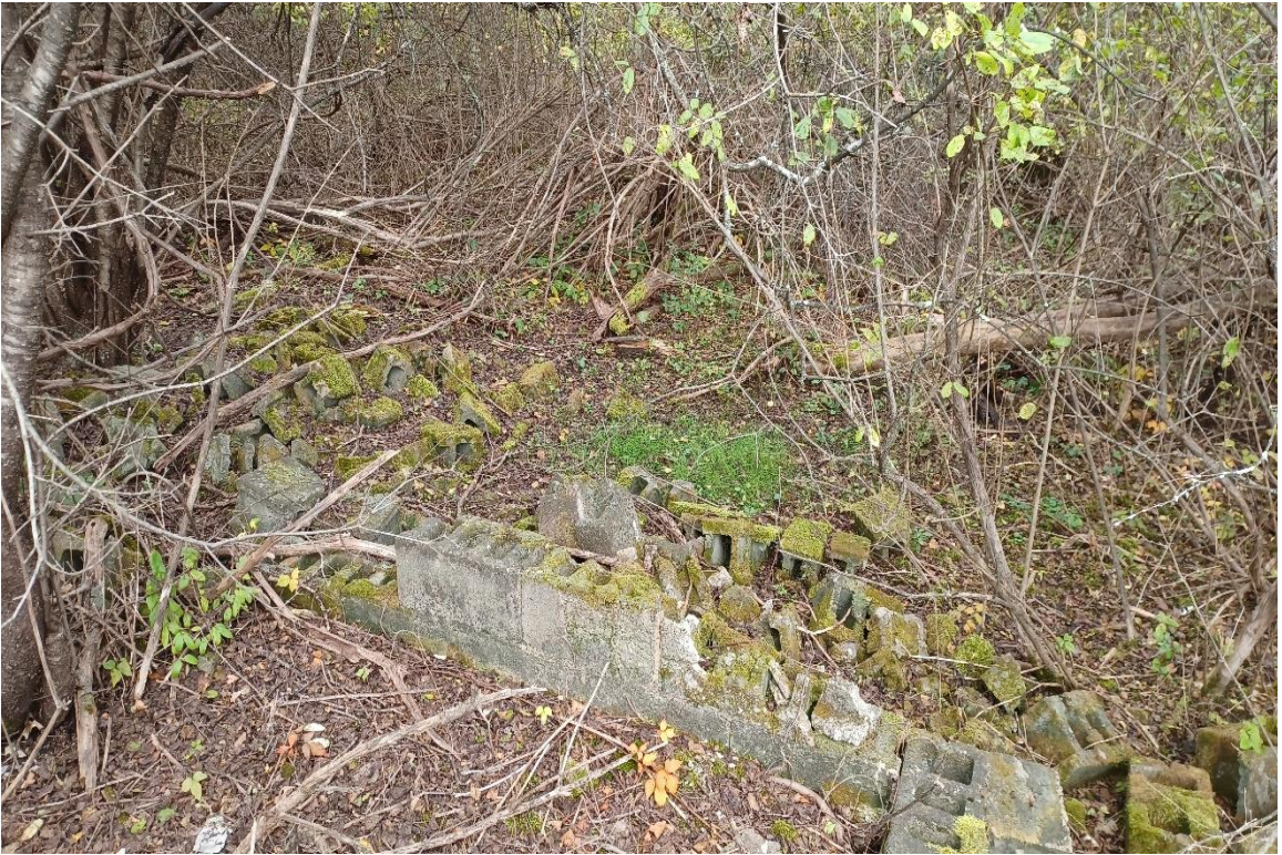
Photo 8: The barn foundation (F4) near the existing silo was constructed of concrete slabs and cinderblock. View to the northwest.
