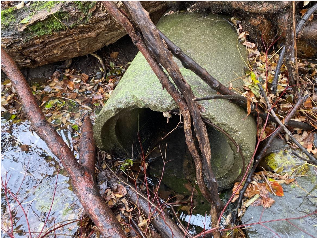
Photo 61: CLV001, inflow. View facing southwest.
