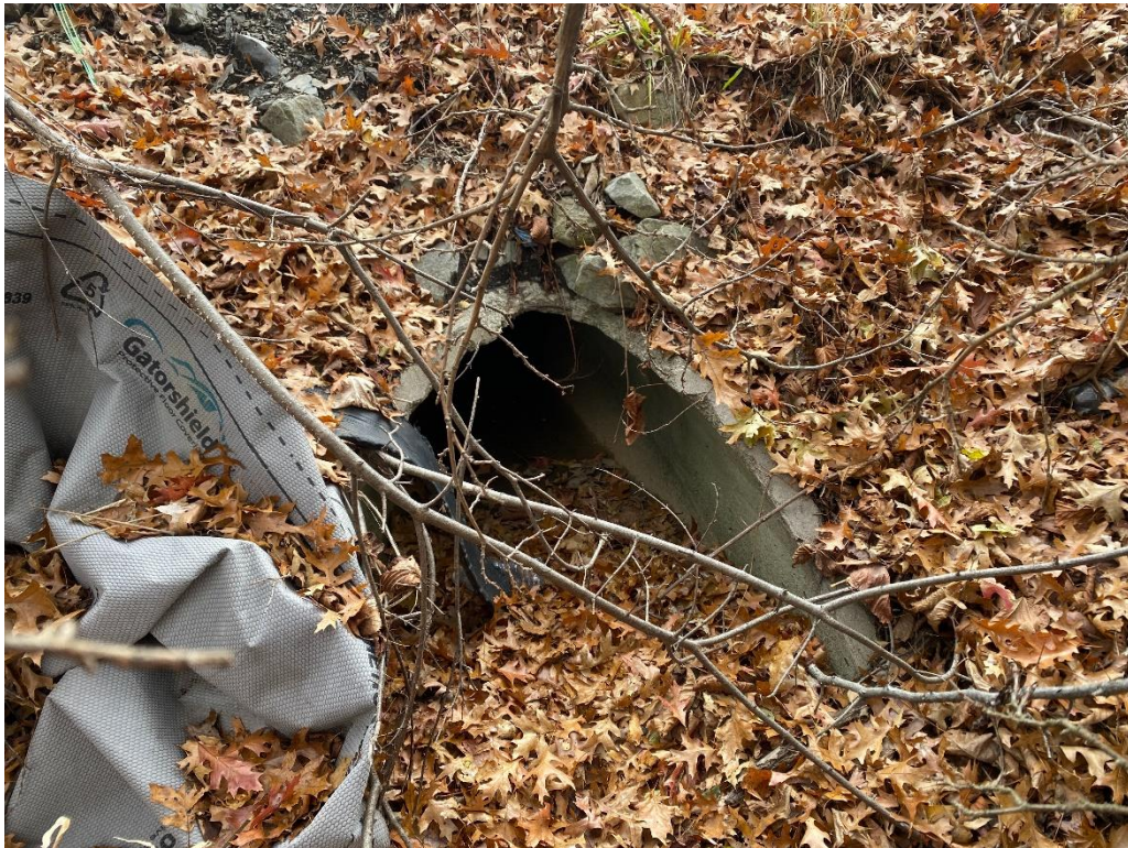
Photo 64: CLV004, outflow. View facing south.
