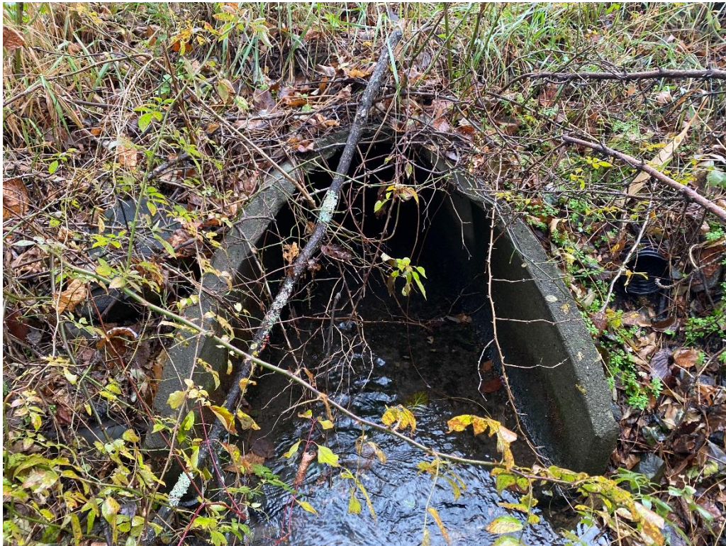
Photo 62: CLV002, outflow. View facing southeast.
