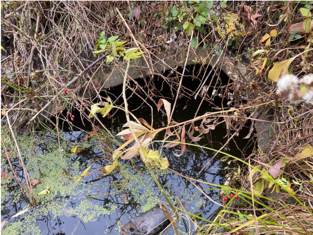
Photo 65: CLV005, inflow. View facing southeast.
