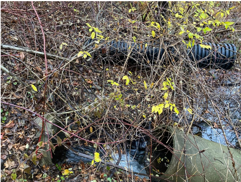
Photo 63: CLV003, outflow. View facing southeast.
