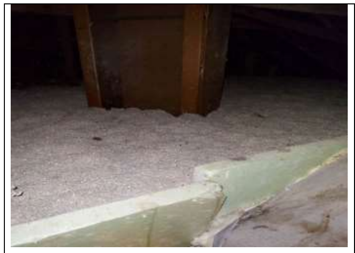
30. View of 497 Beaver Dam Road – Blown-In Attic Insulation
