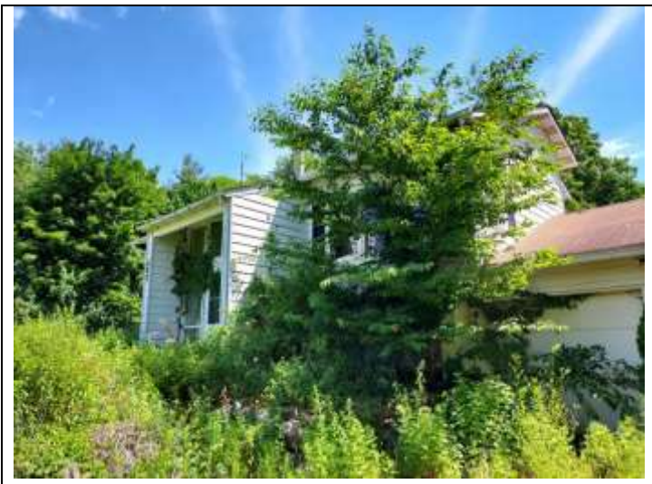
42. View of 483 Beaver Dam Road – Exterior
