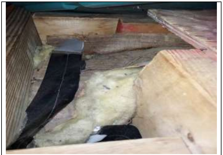
10. View of 355 Neelytown Road - Attic Fiberglass
