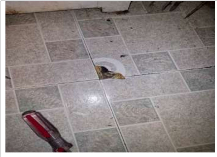
41. View of 475 Beaver Dam Road – Linoleum
