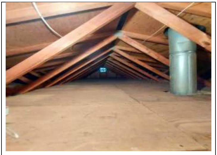
18. View of 497 Beaver Dam Road - Attic
