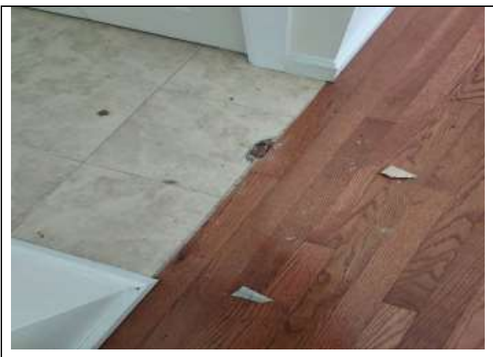
46. View of 483 Beaver Dam Road – Interior Ceramic Tile
