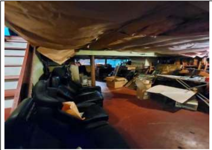
38. View of 475 Beaver Dam Road – Basement
