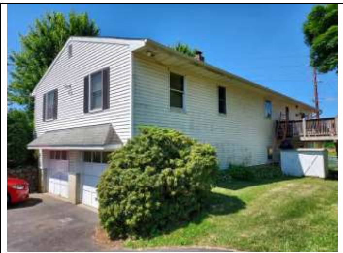
11. View of 497 Beaver Dam Road - Exterior
