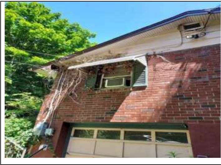
31. View of 475 Beaver Dam Road – Exterior
