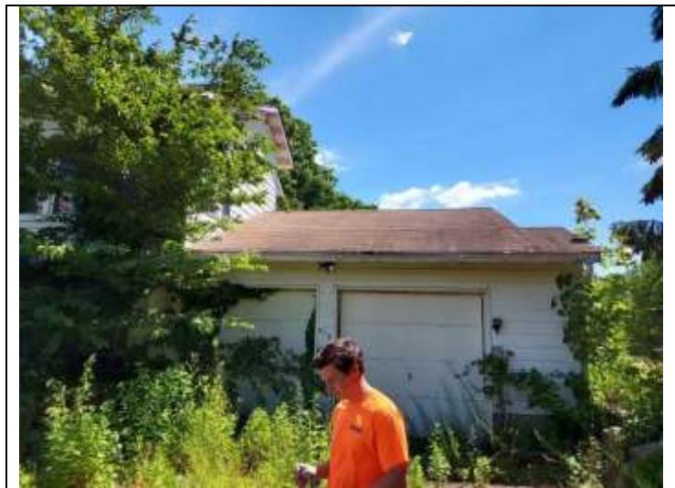
43. View of 483 Beaver Dam Road – Exterior
