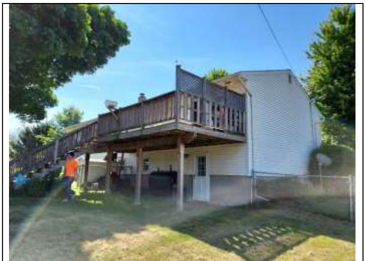
12. View of 497 Beaver Dam Road - Exterior
