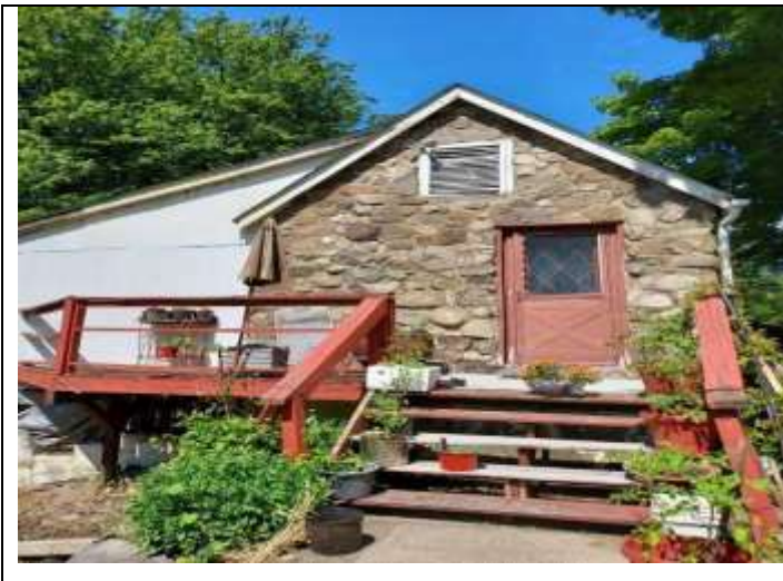
23. View of 497 Beaver Dam Road - Exterior
